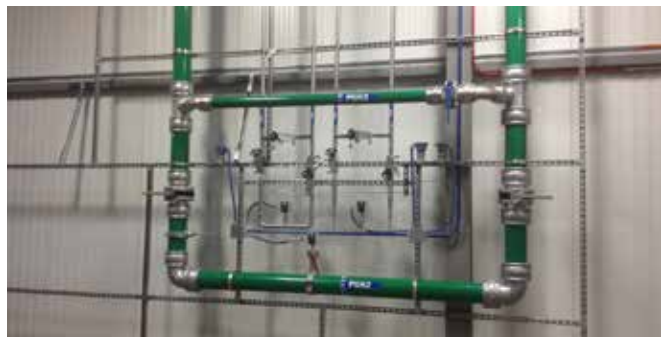
Inert gas Transair® 3" (76 mm)
