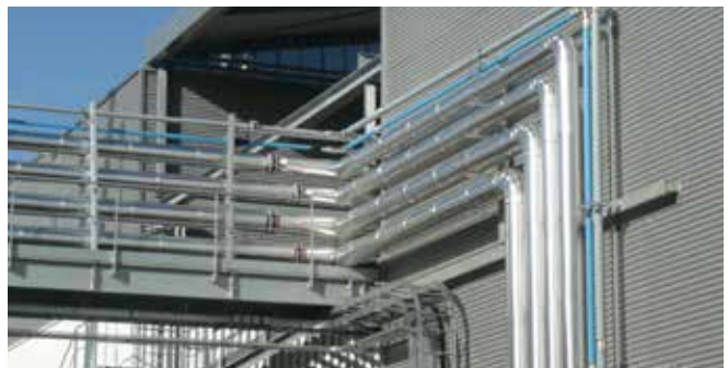
Outdoor installation Transair® 6" (168 mm)
